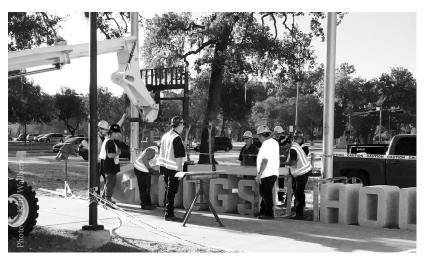
The concrete for the marker was poured in October, followed by the letter and bench installation with the final project being completed in November.
